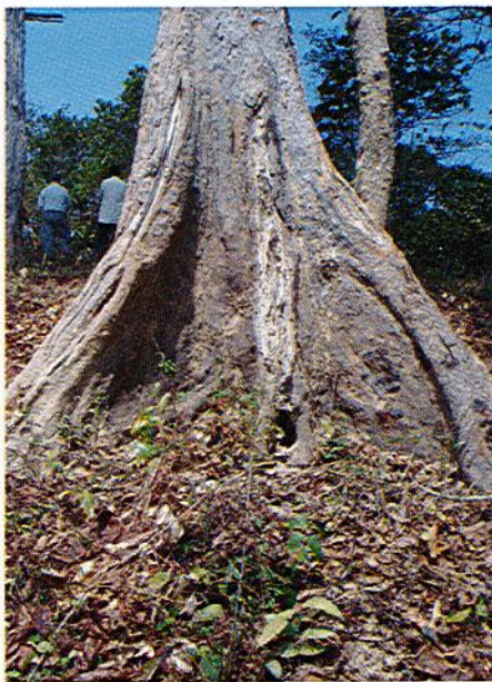
Figure 4. Base of the stem is deteriorating in over-mature trees
