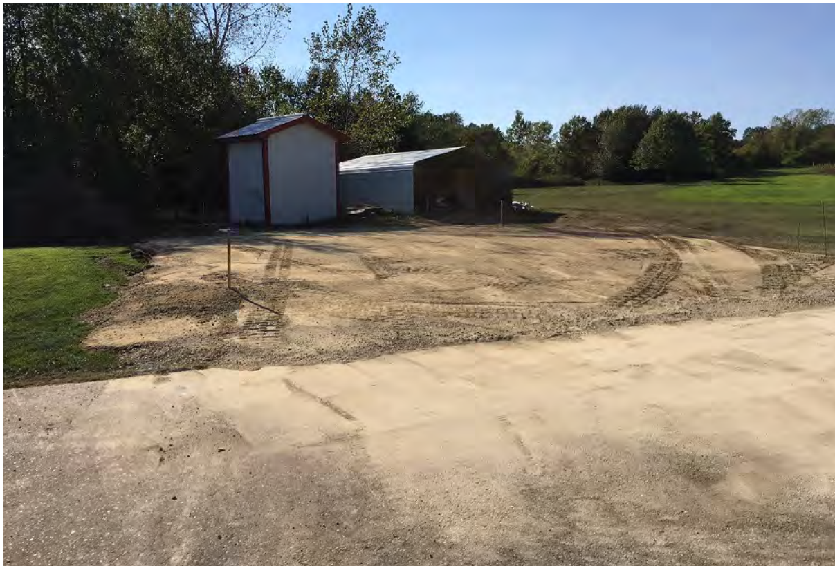
The new pad ready for construction to start.
