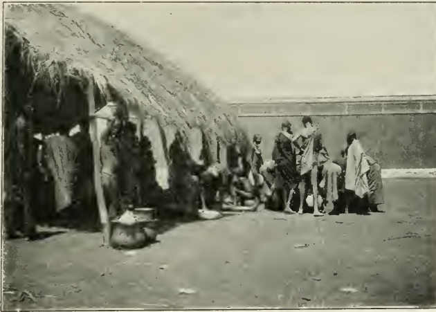
WITHIN THE ENCLOSURE OF THE MARKET, KISUMU.
