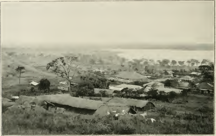
GENERAL VIEW OF ENTEBBE.
