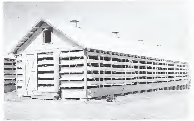
FIGURE 7.—Cone-drying shed, 80 feet long, used by the Southern Region of the U. S. Forest Service.
