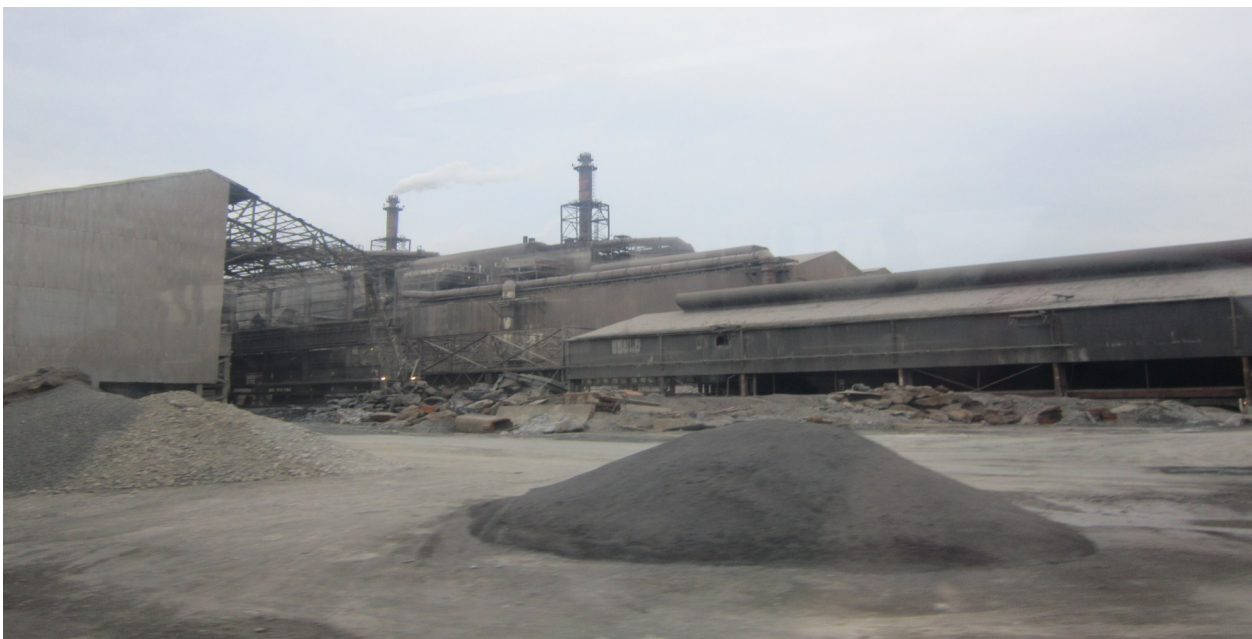
ArcelorMittal Steel plant in Cleveland
