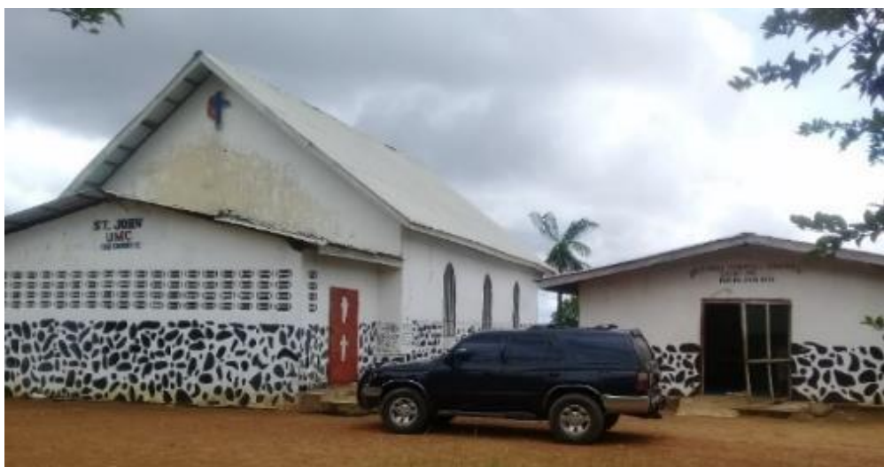
Figure 5-26: A Methodist Church in Plum Hill Community
