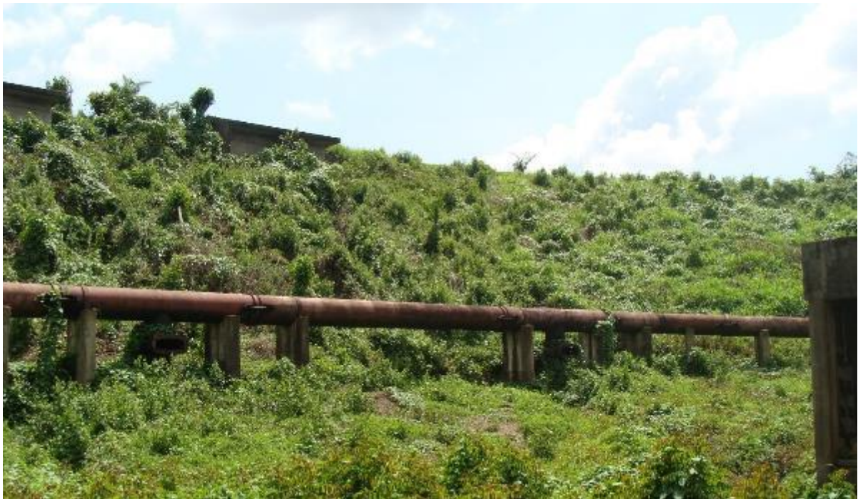
The former Water Transmission Pipeline at MT Coffee HPP in 2011
