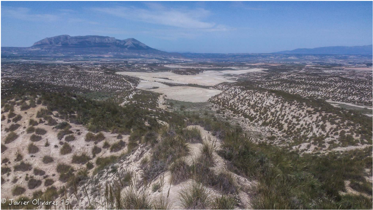
Figure 18. Excavation and trucking on a large area north of Las Hermanillas population of Euchloe bazae in the Hoya de Baza area (photo J Olivares).
