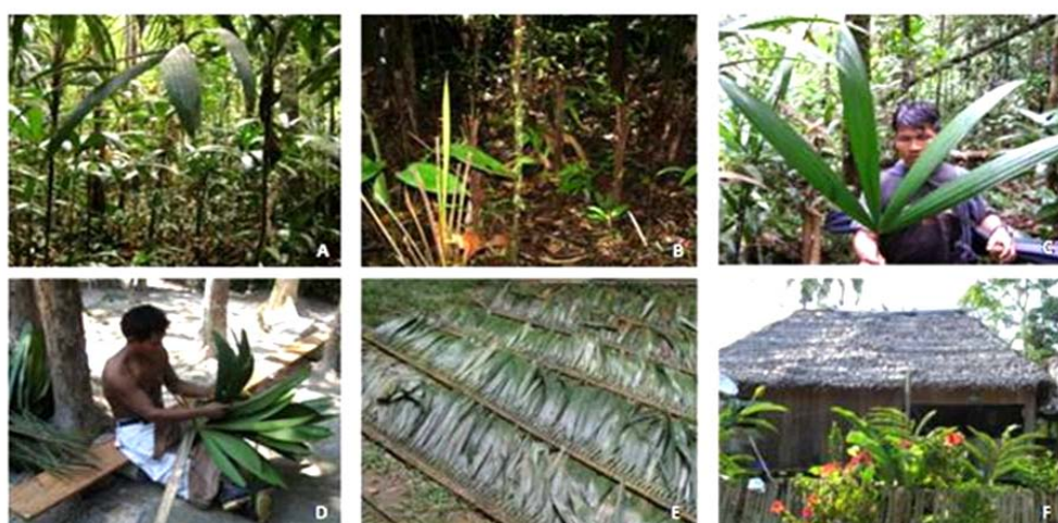
Fig. 8. Different aspects of Lepidocaryum tenue use. (A) Understory of the forest dominated by Lepidocaryum . (B) Lepidocaryum ramets with all leaves cut. (C) Leaves with four segments preferred for thatching. (C) Juan Carlos, an Andoke Indian braiding a Lepidocaryum tile. (D) Lepidocaryum braided tiles finished, (E) House thatch made of Lepidocaryum leaves.
