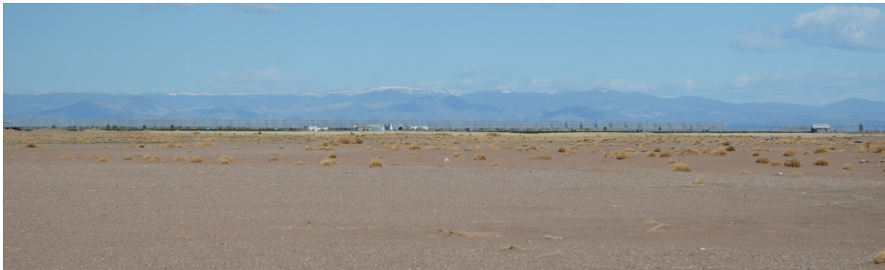
Figure 5.5–4. View of Alamosa Solar Generating Plant, as Seen from a Distance of 2.4 mi (3.8 km).
