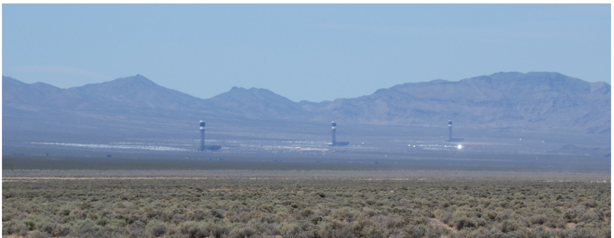
Figure 5.3–6. Glare from Ivanpah Heliostat, as Seen from a Distance of Approximately 11.5 mi (18.5 km), May 2013.
