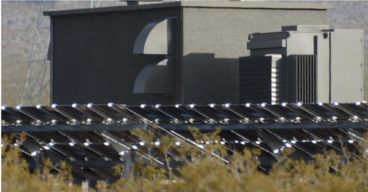
Figure 6.2–6. Sunlight Reflected from the Top Few Inches of the Support Structures Underneath the Solar Panels, and from the Tilt Brackets.
