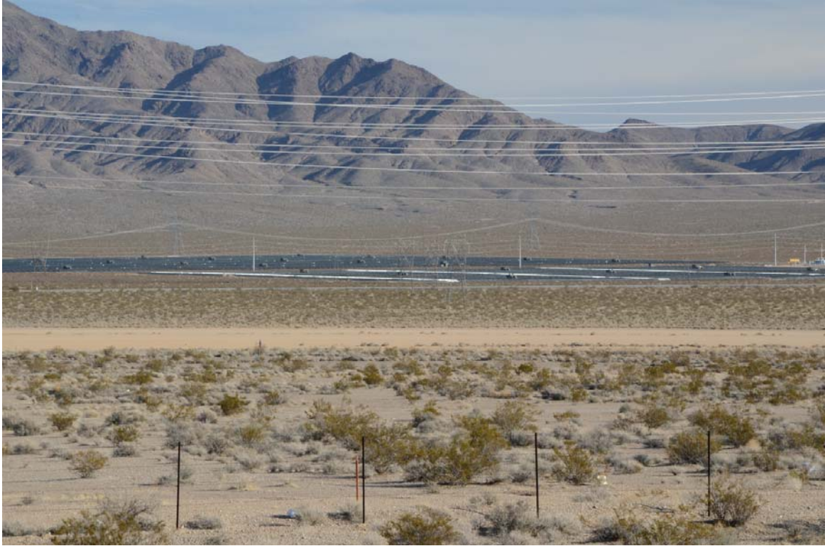
Figure 6.2-7. East-West-Oriented White “Stripes” visible in the Collector Array as Seen from Ground-Level Viewpoint Approximately 1.5 miles from Facility.
