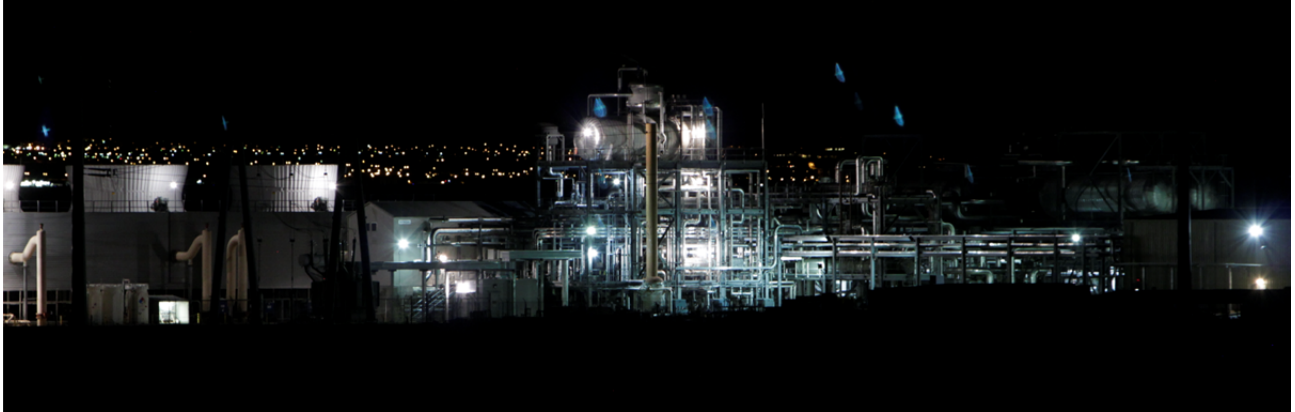
Figure 5.1–5. Nighttime Photo of the Power Block and Part of the Cooling Tower at NSO Parabolic Trough Facility. (Credit: Marc Sanchez, BLM.)
