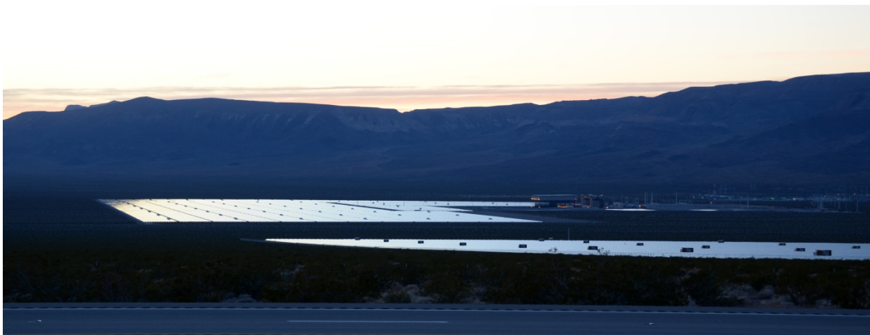
Figure 5.2–1. Black PV Panels at CM 1 and 2 Facilities Appear White When Low-Angle Sunlight Is Reflected from the Panels (Background).
