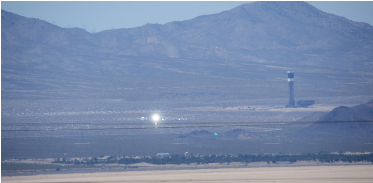
Figure 5.3–5. Close-up View of Glare from Ivanpah Heliostat, as Seen from a Distance of Approximately 10 mi (16 km), May 2013.
