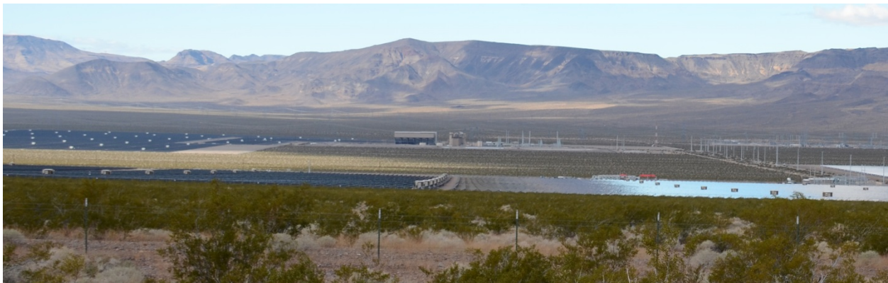
Figure 5.2–3. Brown and White PCUs at CM 2 Facility (Foreground) Contrast with Both Dark (at Left) and Light (at Right) PV Panels. White PCUs of CM 1 Facility Are Visible (Background Left). (Credit: Marc Sanchez, BLM.)
