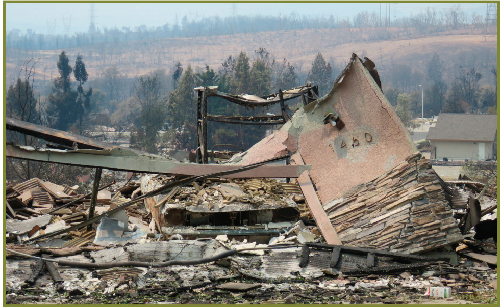
Impact of the Carr Fire, Redding, Shasta County. Photo by: P. Angwin, USFS
