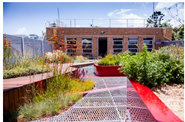
Figure 2.6 Good plant selection is illustrated in the highly diverse plant palette across 14 distinct ‘planting zones’ on the University of Melbourne’s Burnley Demonstration Green Roof. Image: University of Melbourne
