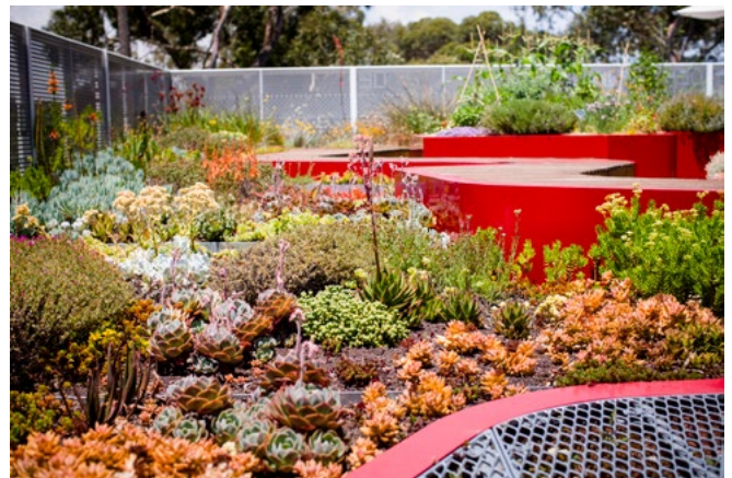
Figure 5.1 Burnley Demonstration Green Roof showing substrate depths and irrigation of different zones. Plants in this case study are found in the 10, 15 and 20 cm unirrigated scoria beds zones 1-3. Images: University of Melbourne.
