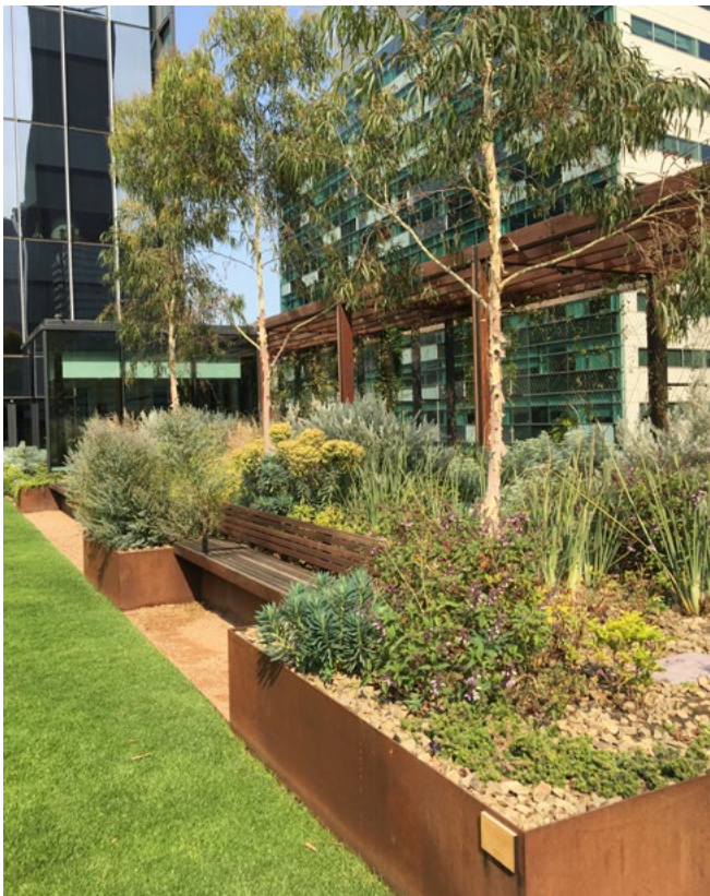
Figure 2.2 A range of engineering solutions can be used to create the required substrate depth and volume to support trees on green roofs, including raised planters (Skypark, Melbourne) and integrated structures (Little Island, New York). Images: R. Bathgate and J. Rayner
