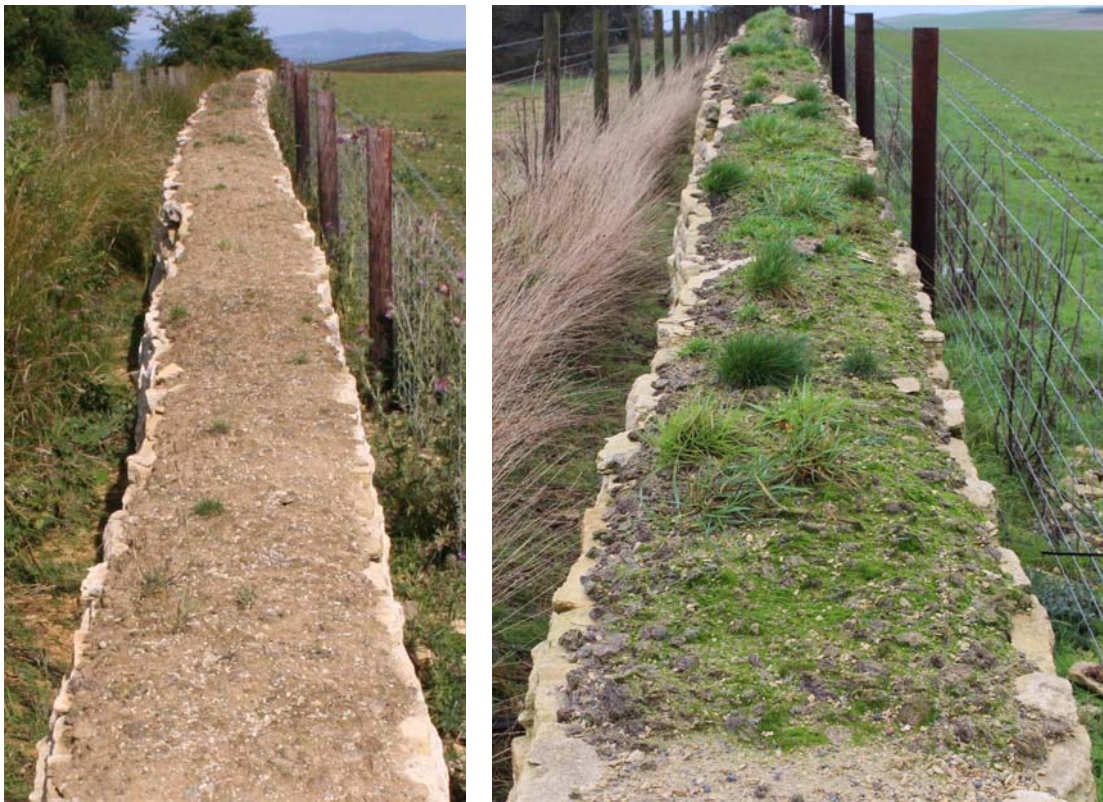
Fig. 1: Colonisation of the mud-capped wall by bryophytes and other plants, in (left) July 2015 and (right) January 2016
