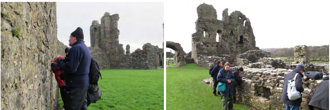
Surveying the walls of Coity Castle (left) and Ogmore Castle (right)
