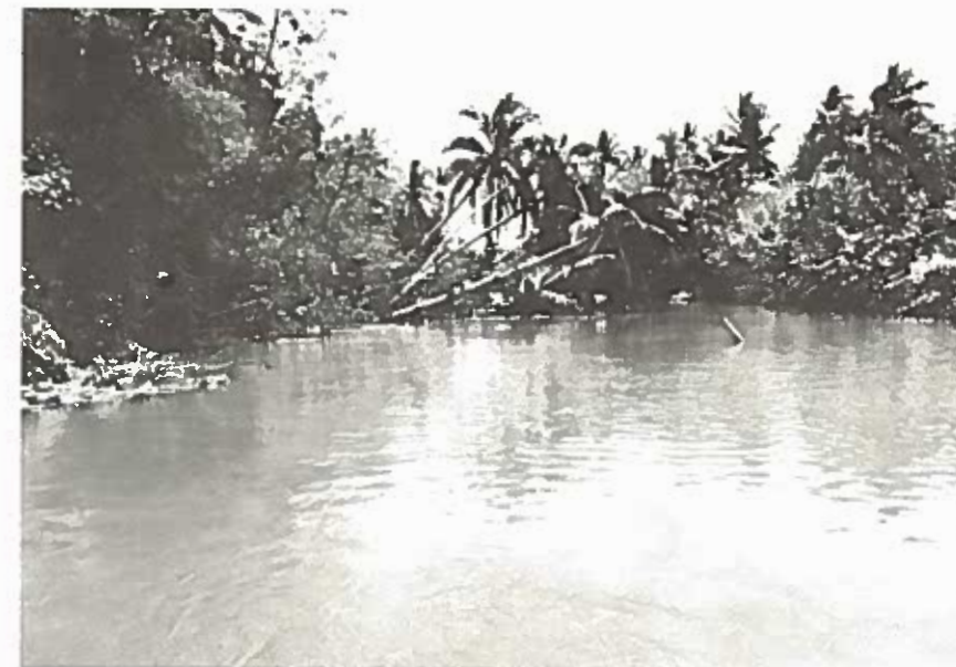
Figure 42. Undercutting and slumping of the alluvial bank along the Talofofu River.
