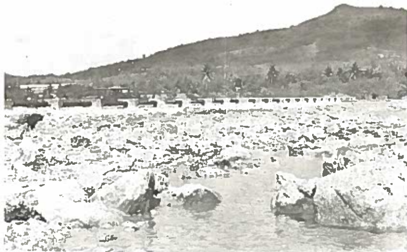
Fig. 38. North side of the peninsula at Gaan Point. Note, the old sewer line running along the top.
