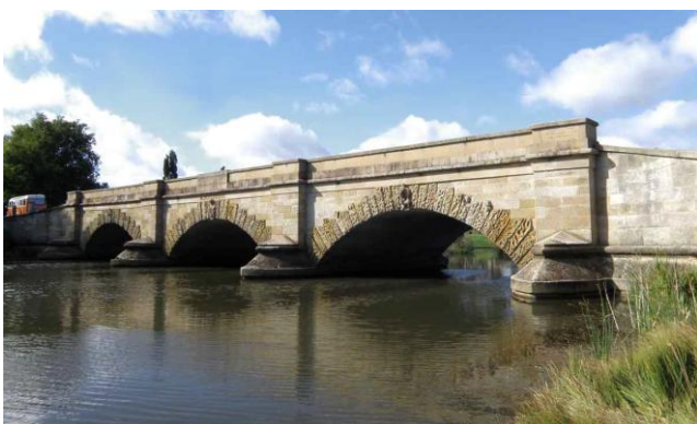
Fig. 15. Macquarie River Bridge, Ross. Photo: JM, 24 March 2012.
