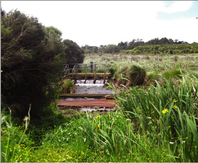
Fig. 3. Waiaatarua Reserve, water outfall, before it flows through a pipe to the Ōrākei Basin, 16 Oct 2017. All photos by Mike Wilcox.
