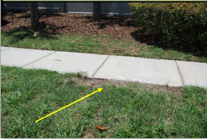
Inbound side of the Glenburne entrance
