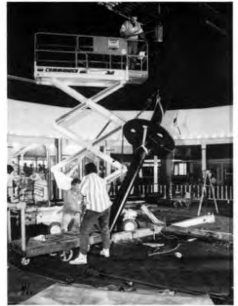
Finally the centerpole is the last piece to be taken down.
