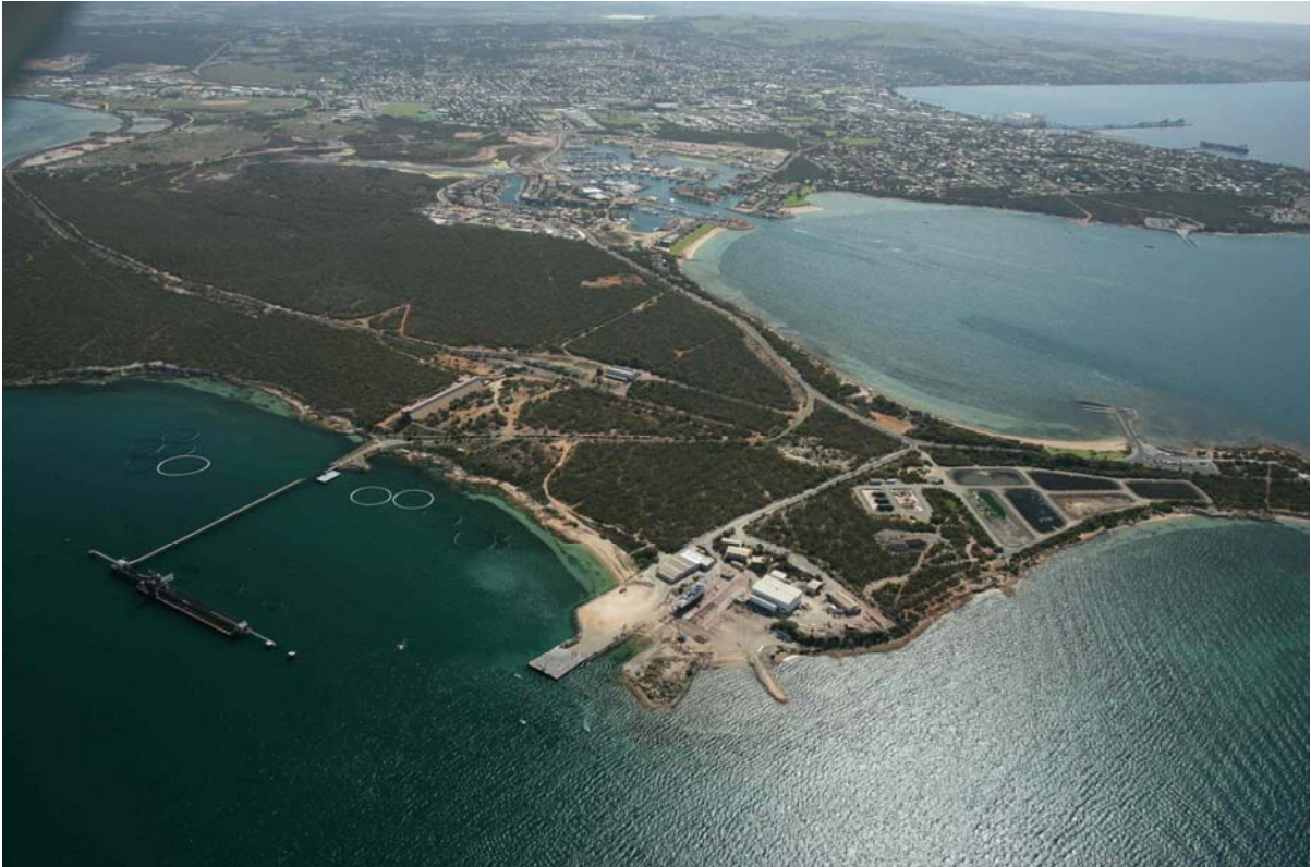
FIGURE 6.11 Billy Lights Point (right), Porter Bay and Lincoln Cove. Photo: Coast Protection Board, 2007
