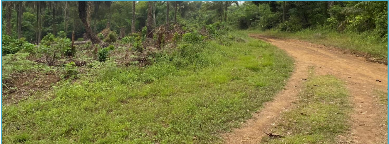
Figure 59: Secondary Gravel Road (Accessing Crawford Farm)
