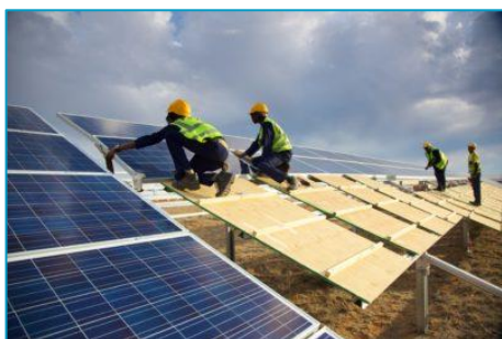
Figure 3. An example of a solar PV plant under construction
