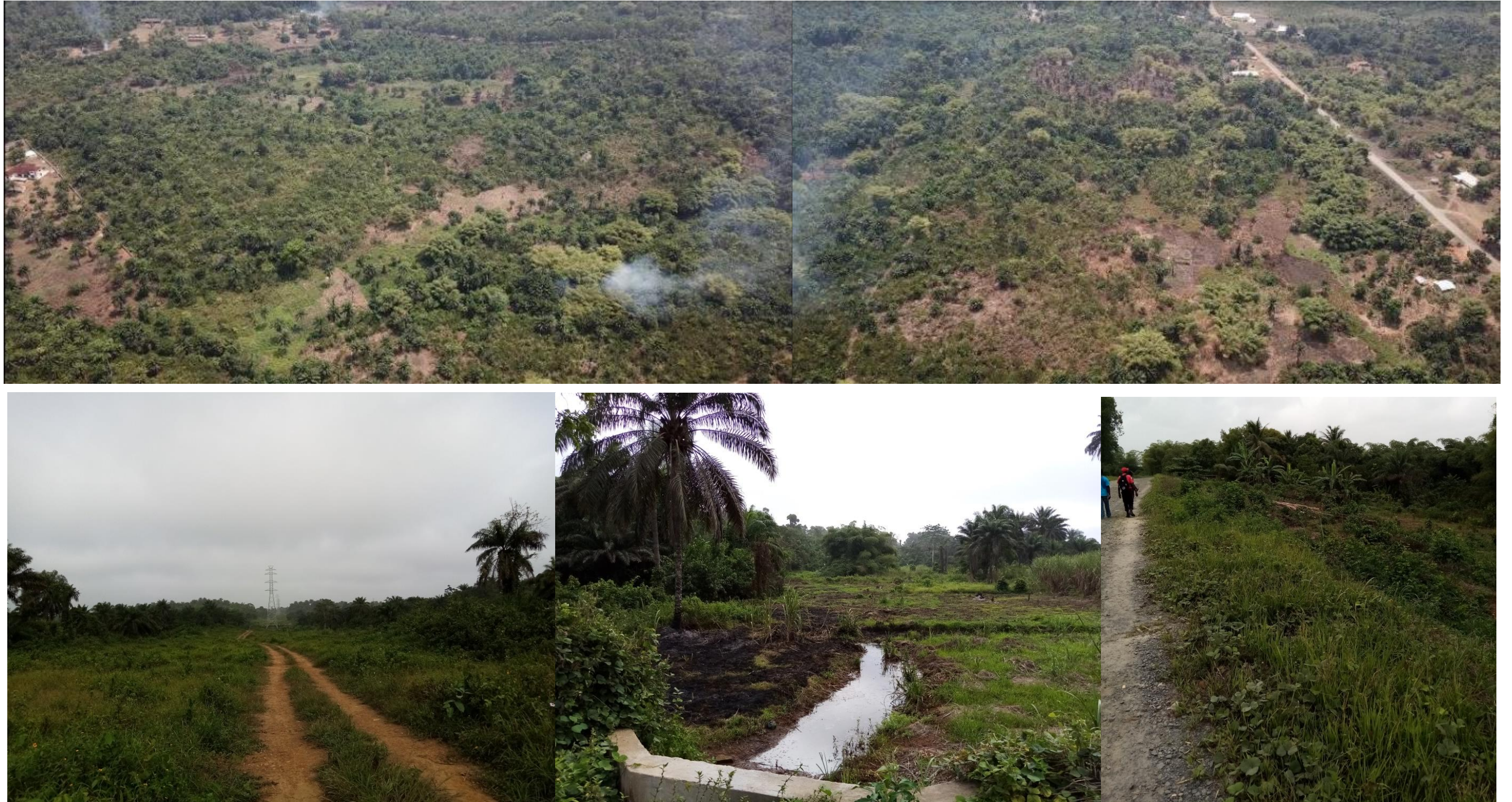
Figure 5: Aerial view (drone footage dated March 2019) and some photos (dated February 2020) of the solar PV site
