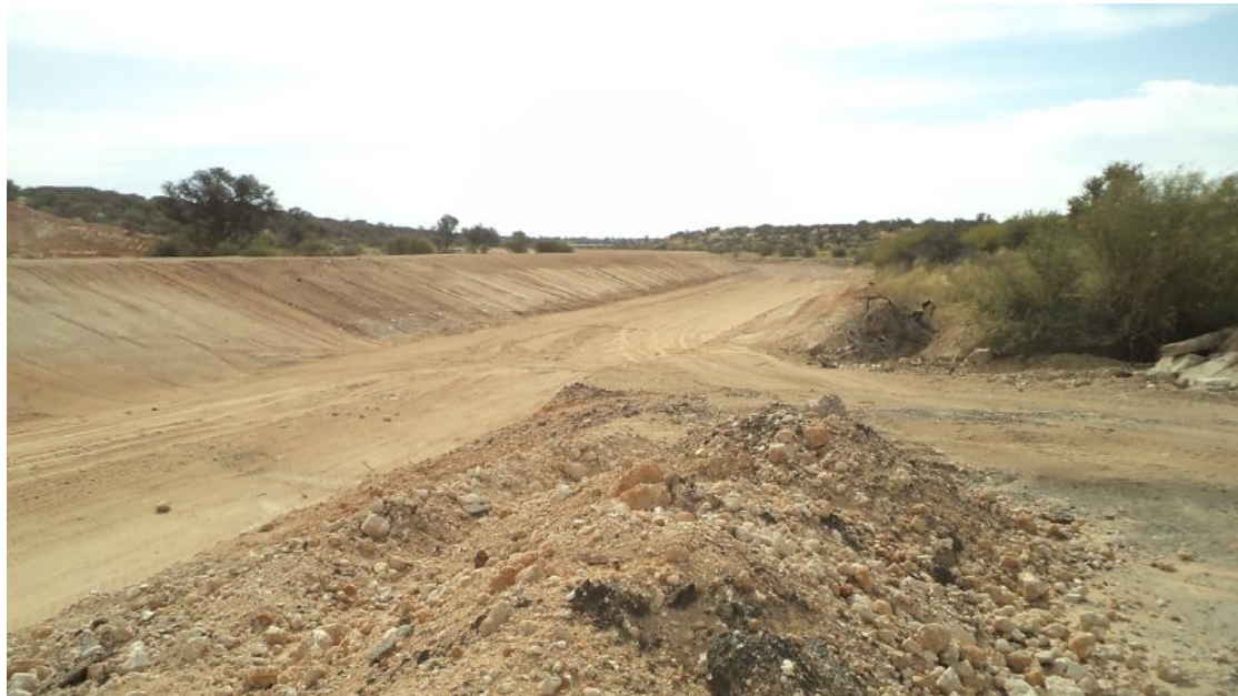
Figure 15 : The area of the river channel diversion
