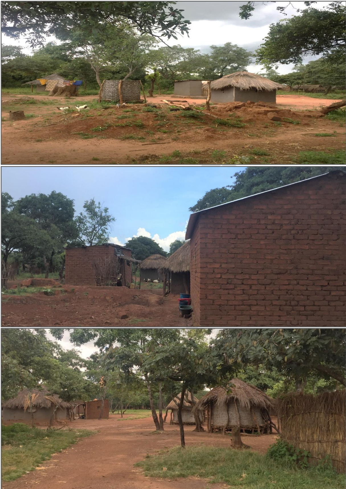
Figure 20: Typical Examples of homesteads and related structures
