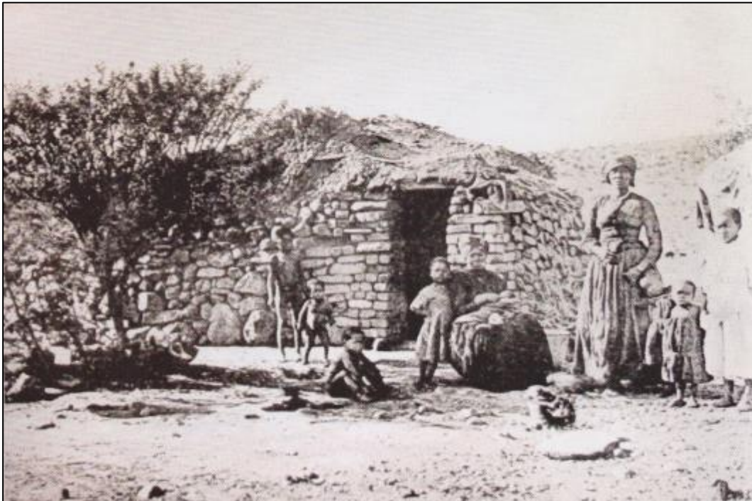
Figure 7-81: A shepherd's hut photographed near Beaufort West in the early 20th century. Note the low, narrow doorway and informal roof structure. Source: Schoeman (2013:48)
