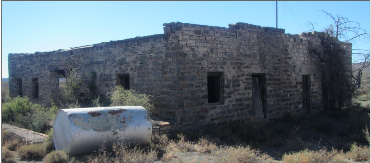
Figure 7-98: A derelict outbuilding alongside the main house at waypoint 1791 in HL04.
