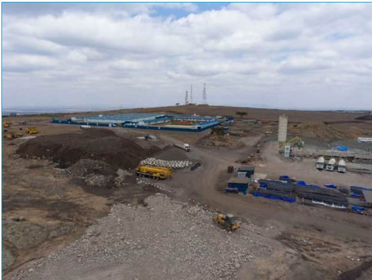
Figure 14: Example of General laydown area and construction camp 3
