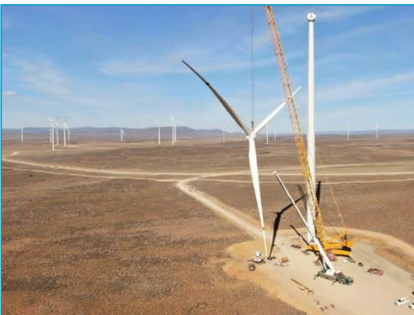
Figure 4. An example of a wind turbine under construction
