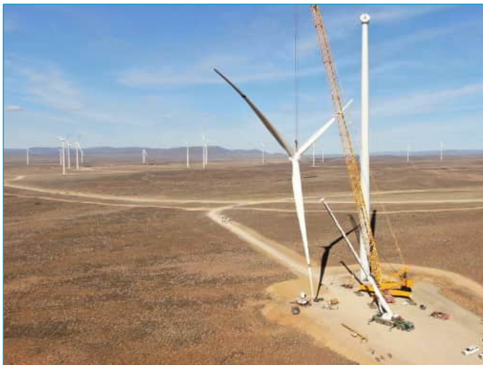
Figure 20: Example of wind turbine under construction 6
