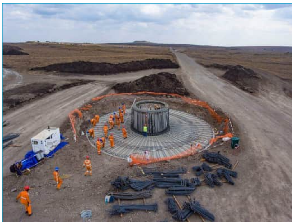
Figure 16: Typical wind turbine foundation
