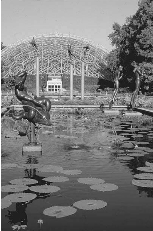
Figure 5.7 Climatron® at the Missouri Botanical Garden, a Geodesic dome with Climatic control and supporting tropical rainforest. (Photograph by Jack Jennings/Courtesy the Missouri Botanical Garden).
