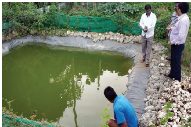
Plate 48: Rainwater harvesting in the lined ponds at Car Nicobar
