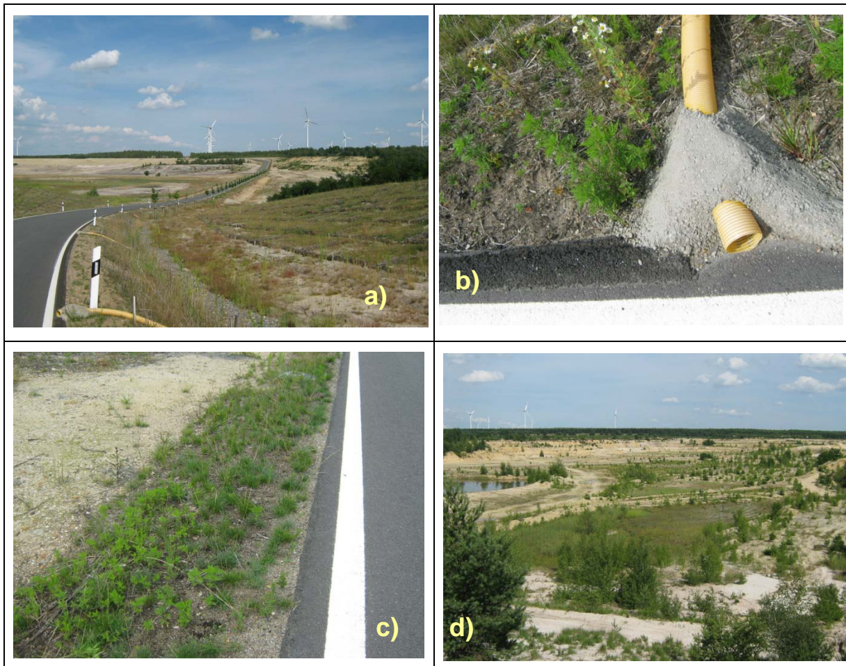
Fig 15: Newly built road in a reconstruction area connecting the villages Klettwitz and Kostebrau near Senftenberg (photo: 2011/07/06).
