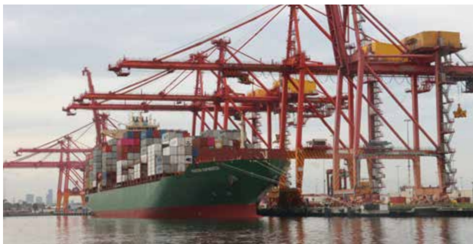
Access to reliable shipping routes, freight and logistics will most certainly represent challenges for the foreseeable future.
