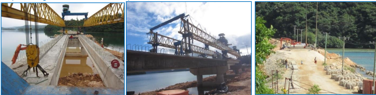
Vaipua Bridge Reconstruction Completed to December, 2012.
