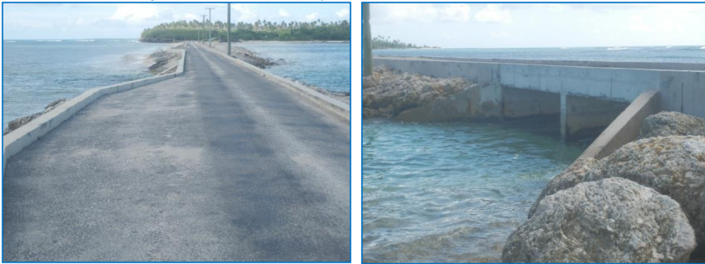
Foa Causeway Rehabilitated Completed to December 2013.
