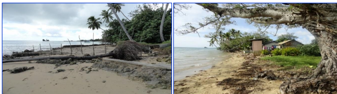
Severe erosions at Lifuka Island.
