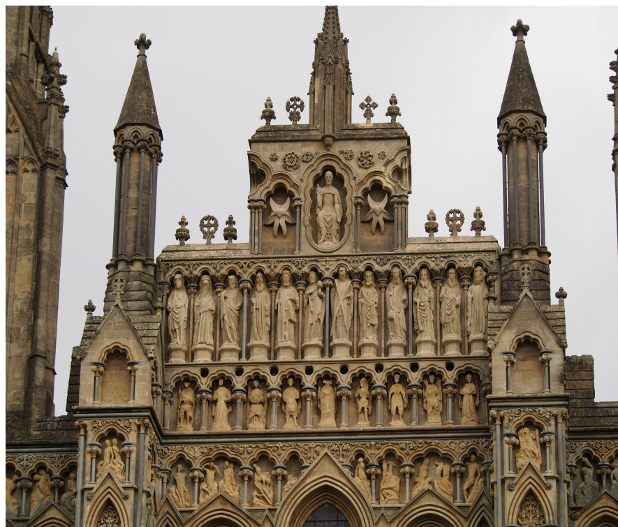
Figure 12: The completed works
