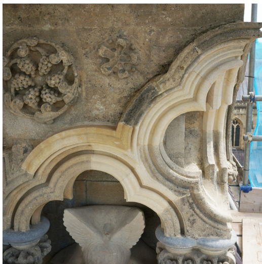
Figure 8: Completed stone repairs to quatrefoil
