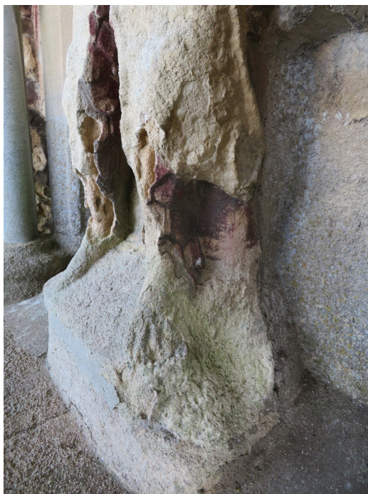
Figure 3: Typical blistering patterns and loss of structure to form
