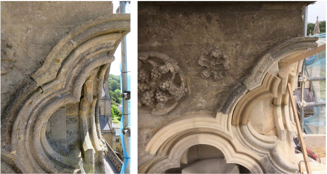
Figure 7: Quatrefoil section before and during works
