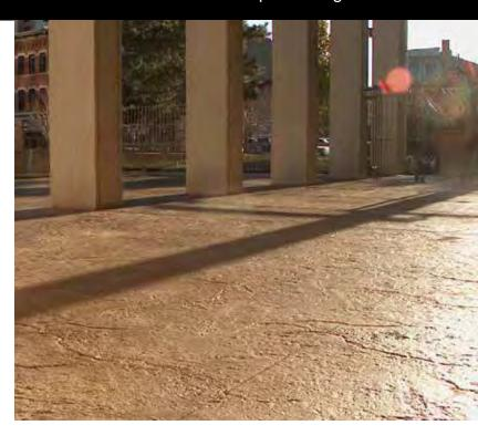
Brickform Stampable Overlay "Gray" is a premixed blend of special materials that, when mixed with water, forms a thin, concrete coating. This overlay is intended for use with Color Hardener and Antique Release.
