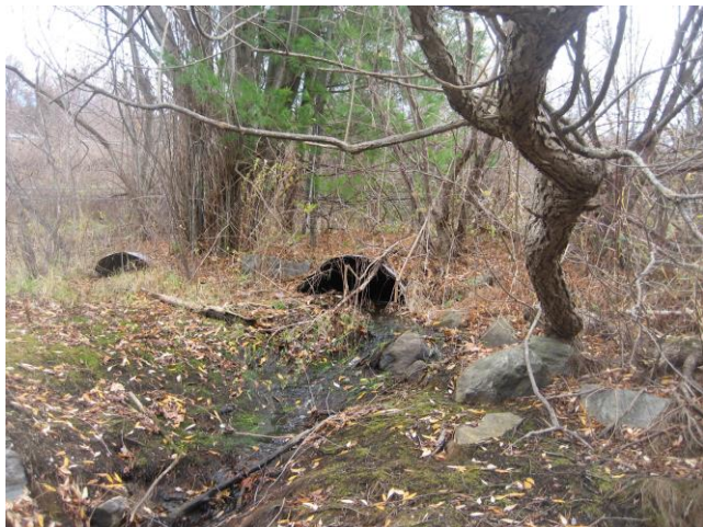
3 culverts beneath Byram Lake Road at BLT 2, looking east
