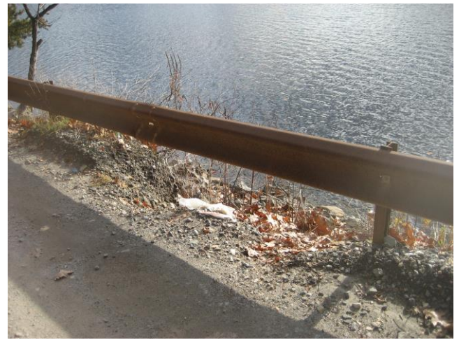
Eroded embankment along Byram Lake Road at north end of lake
