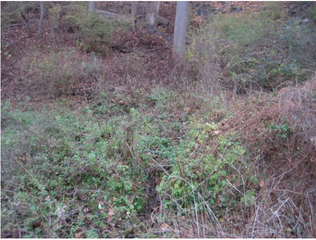
Hillside stream and check dam with culvert
