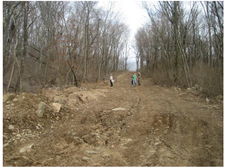
Erosion along water tower road
