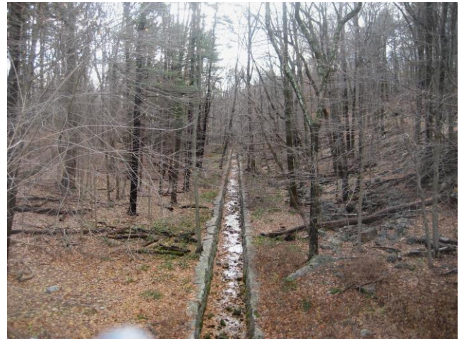
Byram River beneath dam/lake
