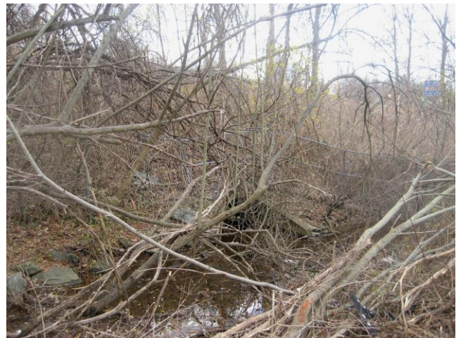
Further upstream looking east to culvert beneath highway
