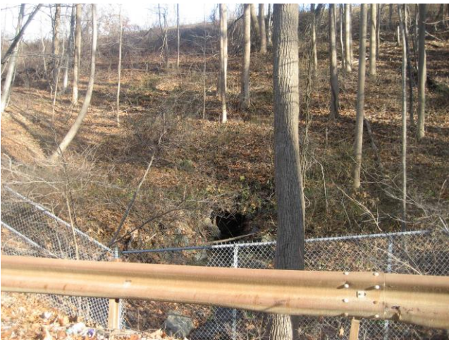
Culvert looking east at steep slope and highway
