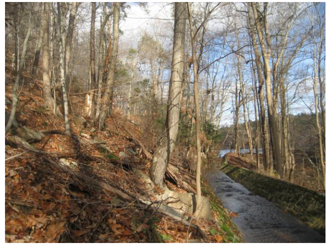
Sluiceway with vegetated steep slope to west
