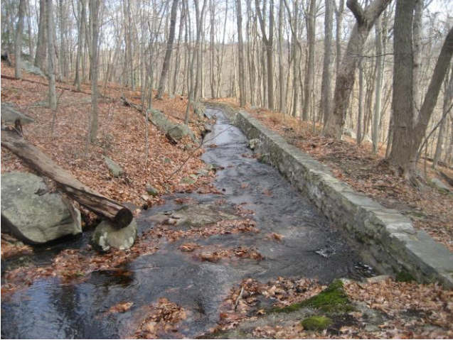
Stream re-directed into sluiceway
