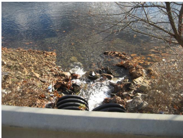
Culverts emptying marsh into Byram Lake from beneath Byram Lake Road
