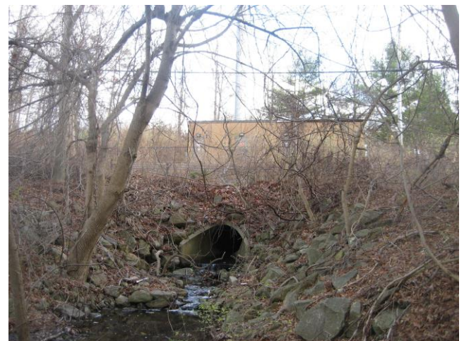
Concrete culvert at BLT 4 with cell tower across Byram Lake Road
