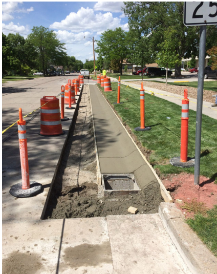
18th Street & 3rd Avenue
