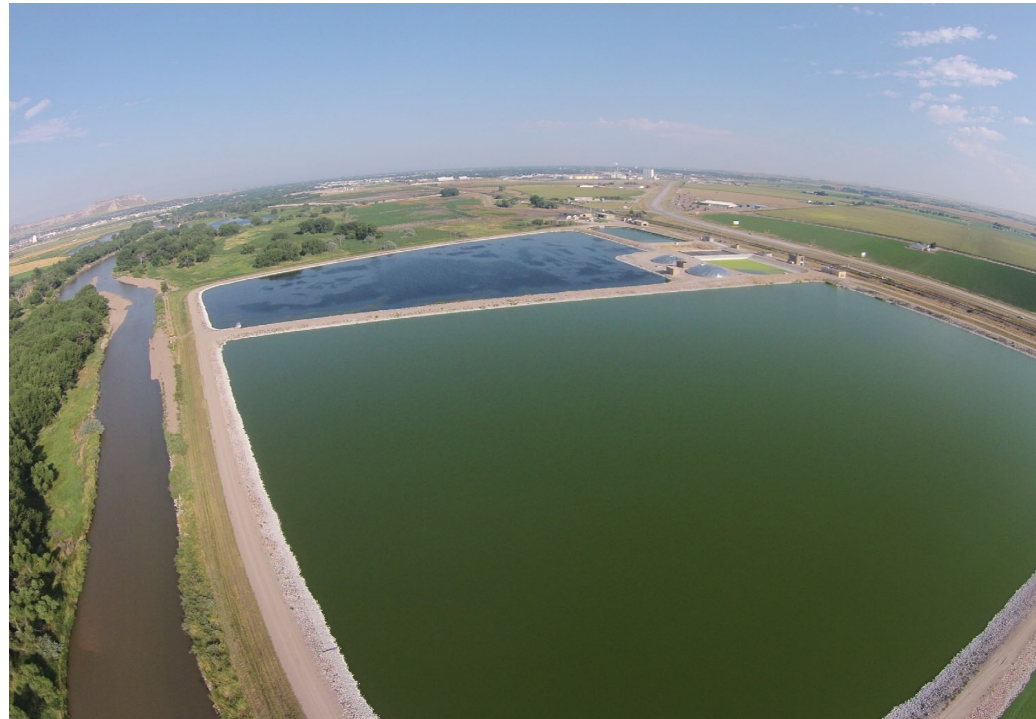
City of Scottsbluff, Wastewater Treatment Plant
