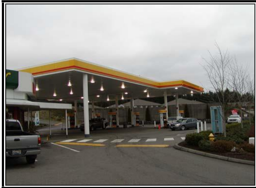
Figure IV-6.3 Roof at Fueling Island to Prevent Stormwater Run-on.
