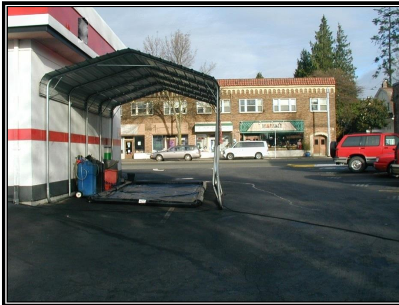
Figure IV-5.1 Wash Pad for Tool and Equipment Washing
