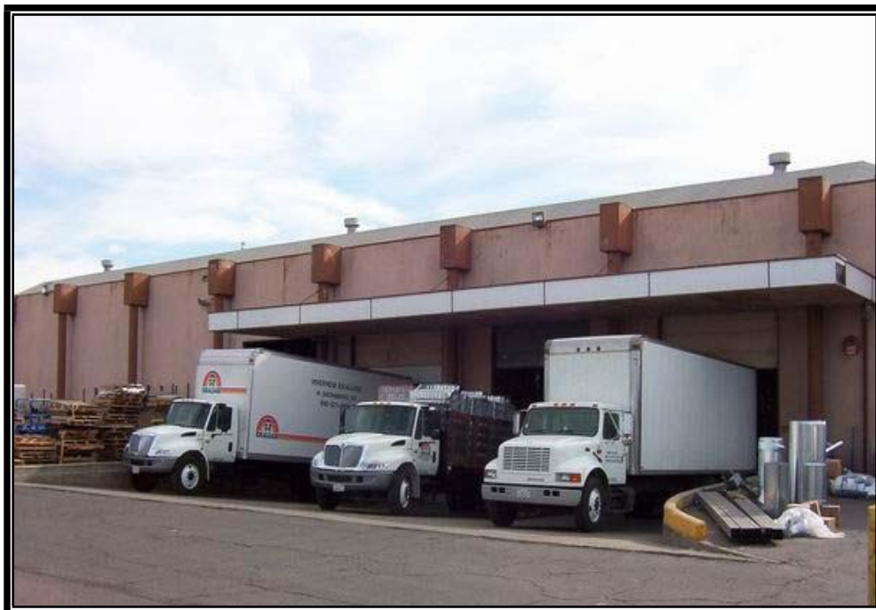
Figure IV-6.2 Loading Docks with an Overhang to Prevent Material Contact with Rainwater.
