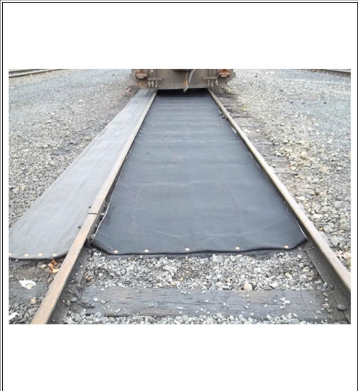
Figure IV-5.16: Installed Railroad Track Mats
