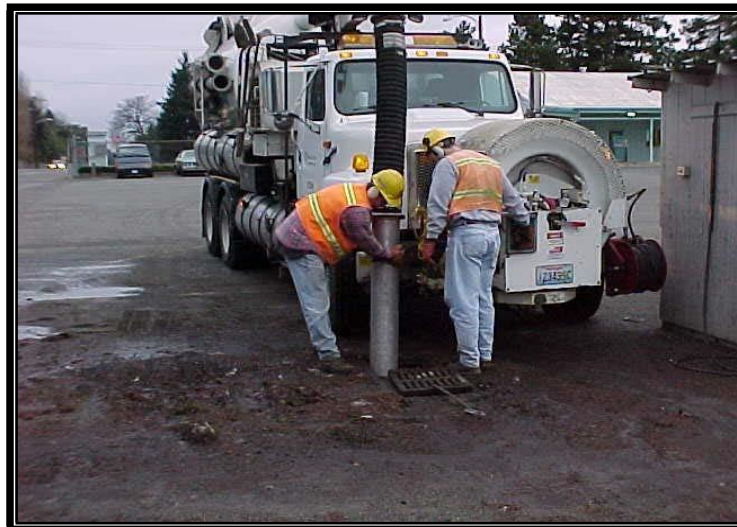
Figure IV-6.8 Catch Basin Cleaning with a Vacuum Truck.
