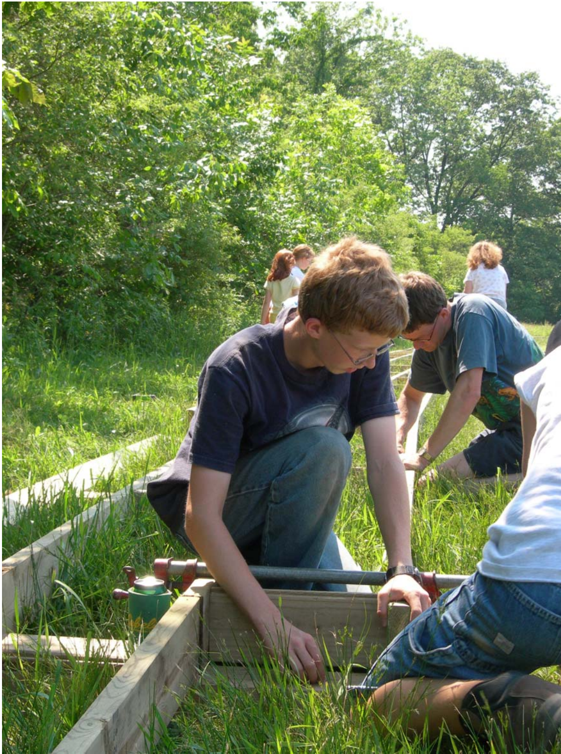
OWC NERR volunteers assemble a boardwalk section
