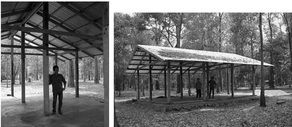
Figure 7. The public hall under construction
