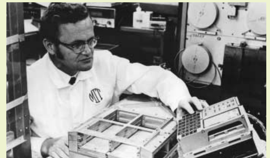
Lead designer Eldon Hall testing the Apollo Guidance Computer
