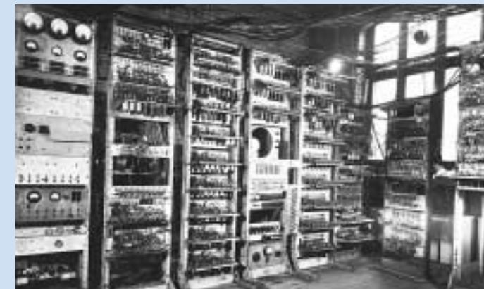
While working for Williams, Kilburn and Tootill built the Baby to demonstrate the viability of CRTs for storage (memory). It worked successfully for the first time on June 21, 1948, becoming the world's first functioning stored program electronic computer.
