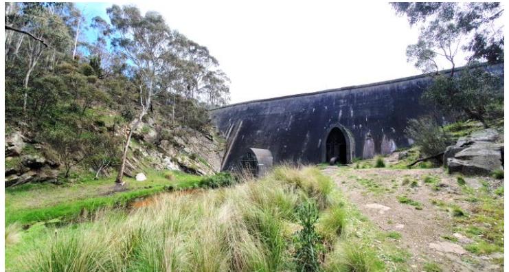
Base of the Lower Stony Creek Reservoir (Photo: Tamara Leitch)
