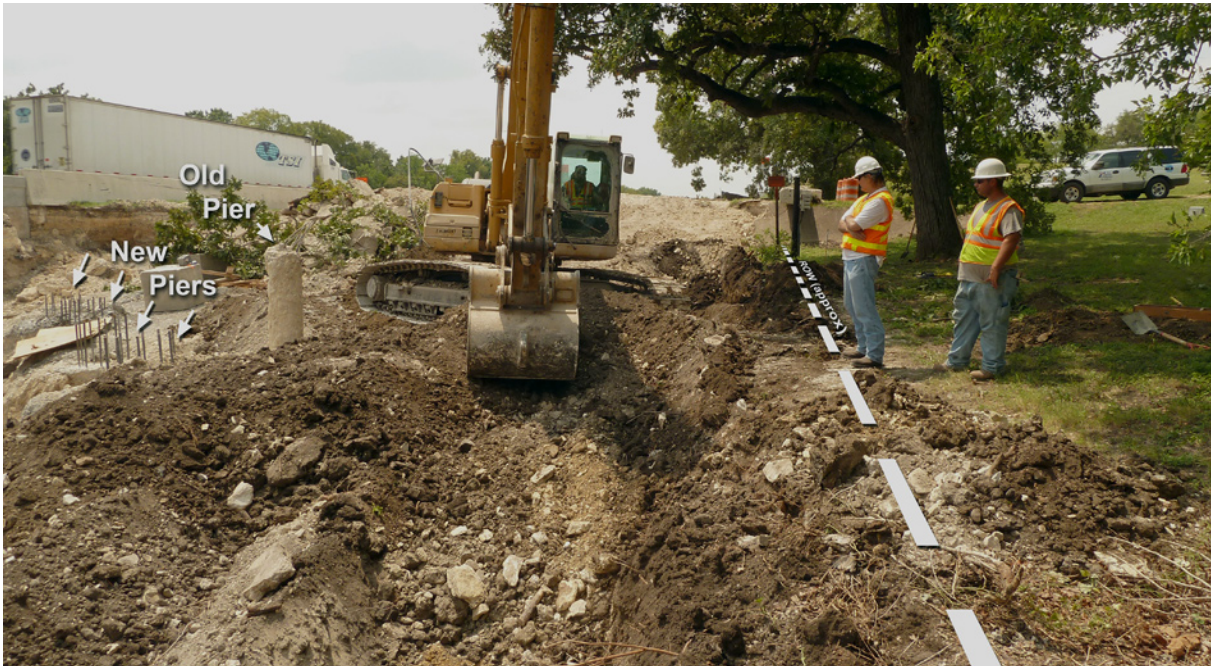
Figure 2.4. View of trenching showing the character of the rubble fill.
