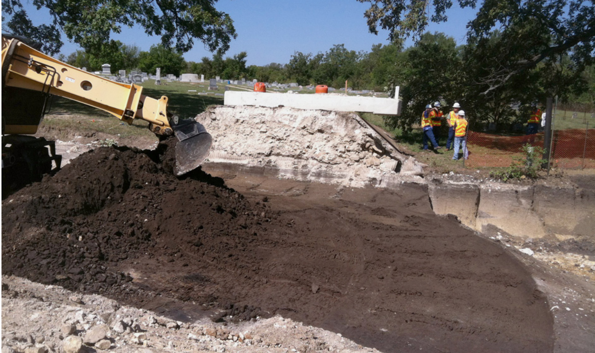
Figure 2.10. Systematic stripping of the A horizon beneath the frontage road fill section, looking west. Note the trapezoidal rubble fill section of the former cemetery entrance ramp in middle ground.
