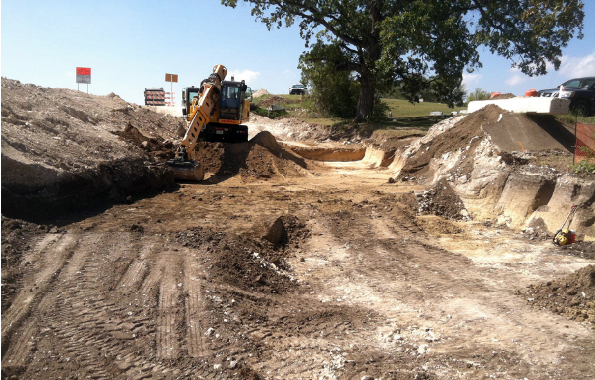
Figure 2.11. Systematic stripping of the lower B and C horizons, looking south.
