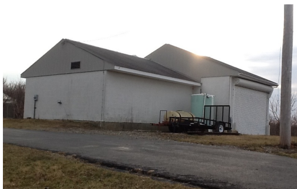
Pesticide Storage Building with water tank in current position next to the building, and new, black utility trailer in the foreground
