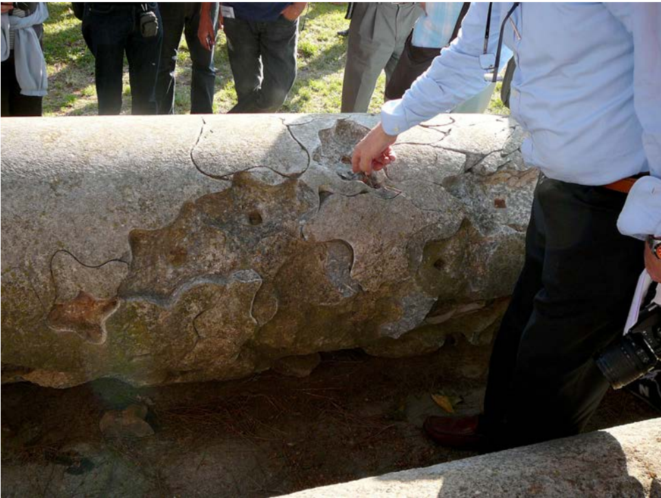
Fig. 11: Method of interventions and repairs of ancient stonemasons into the shafts of the columns left in the statio marmorum from the Ostia/Portus area, now in the open-air museum of Parco archeologico di Ostia antica. Photo by H. Tůmová.
