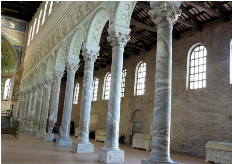
Fig. 9: Monolithic marble columns, bases, and capitals ‘a foglie d’acanto mosse dal vento’ in the basilica of San Apollinare in Classe (Ravenna). Photo by H. Tůmová.
