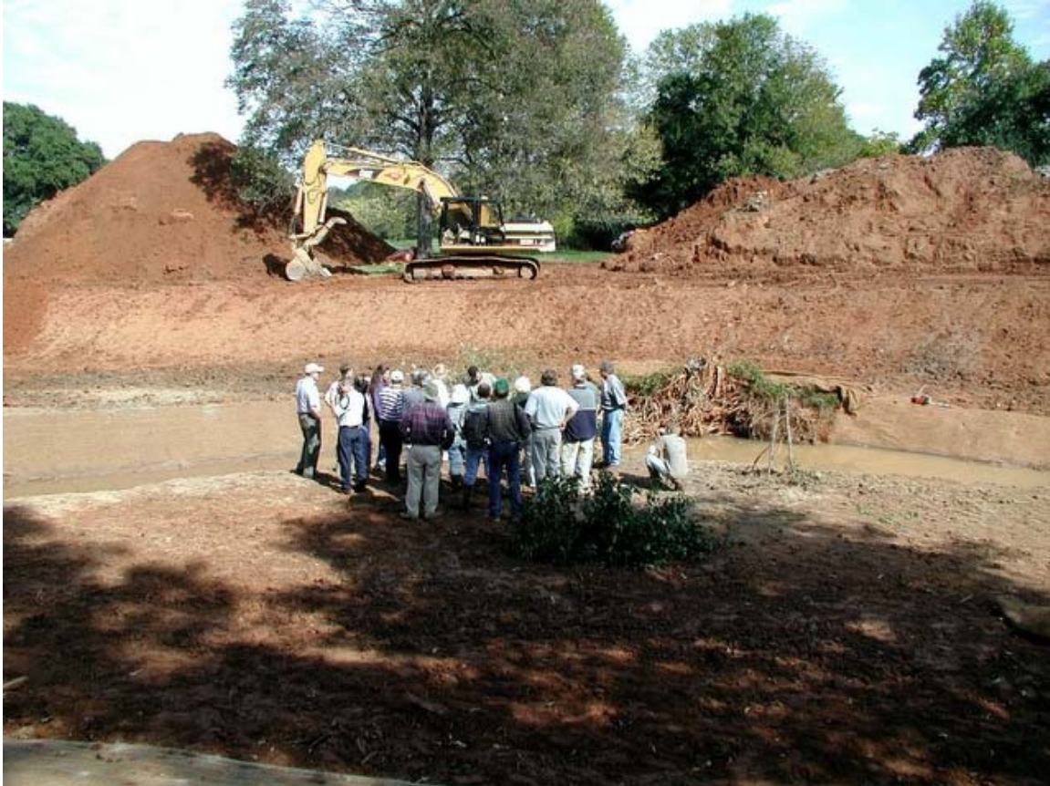
Figure 16: Stream restoration on Clemson University property.
