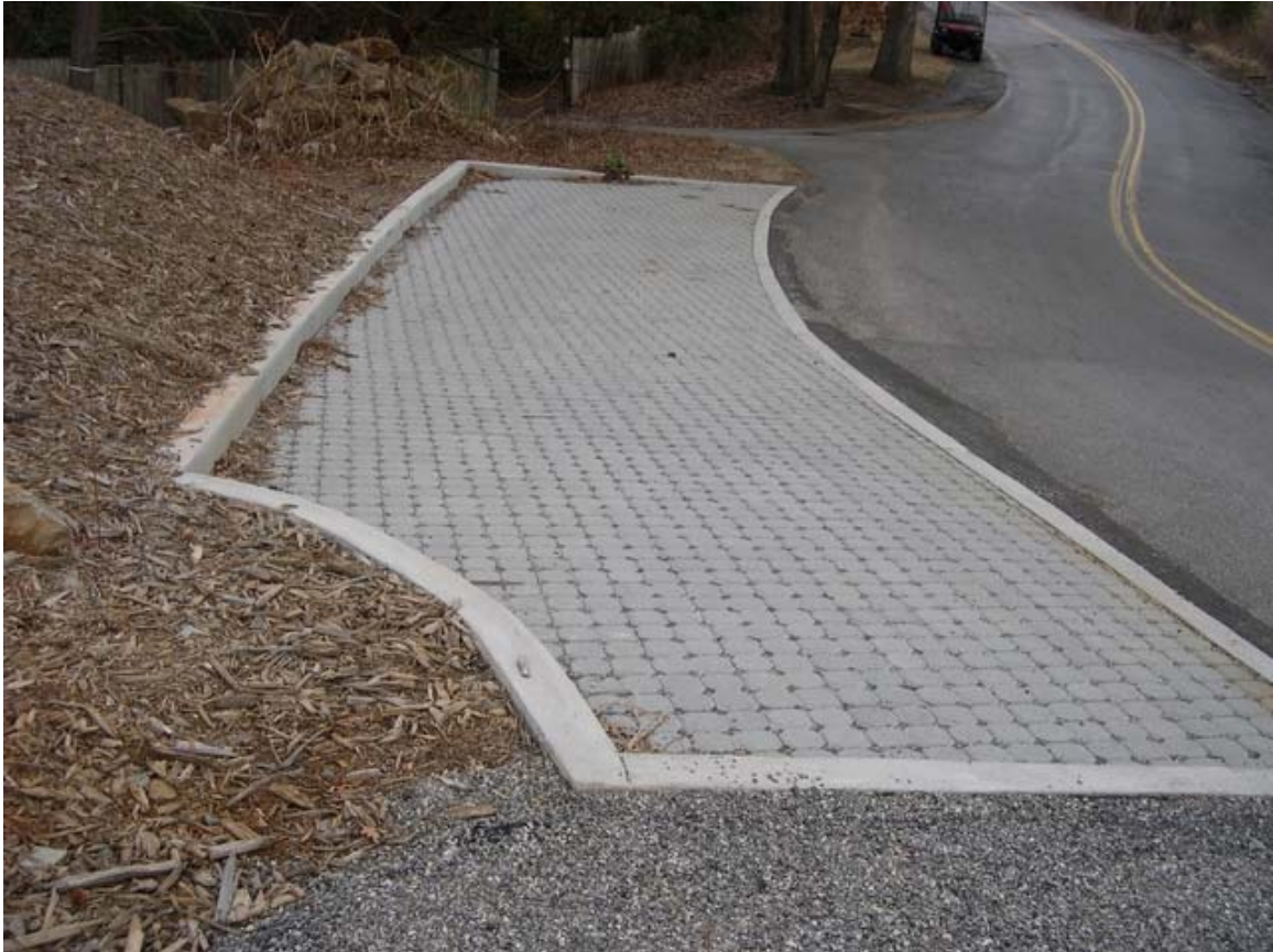
Figure 14: Permeable Paving for Bus Parking.
