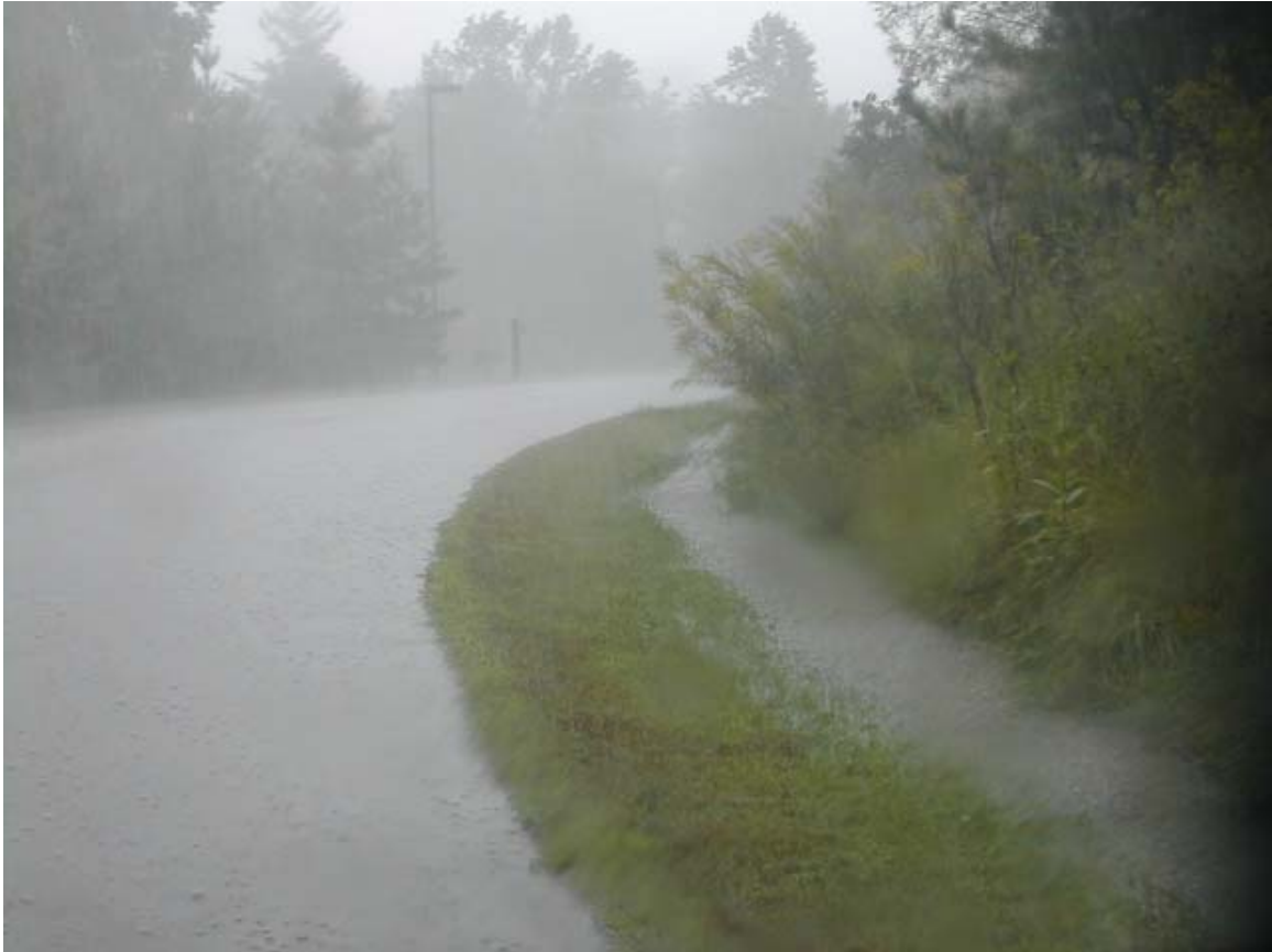
Figure 13: Turf Reinforced Swale conveying runoff.
