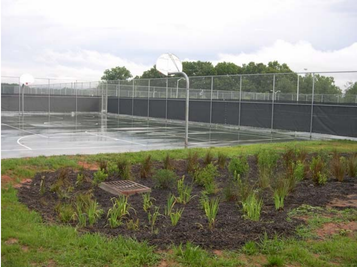
Figure 11: Rain Garden treating runoff at Asheville Buncombe Technical College.
