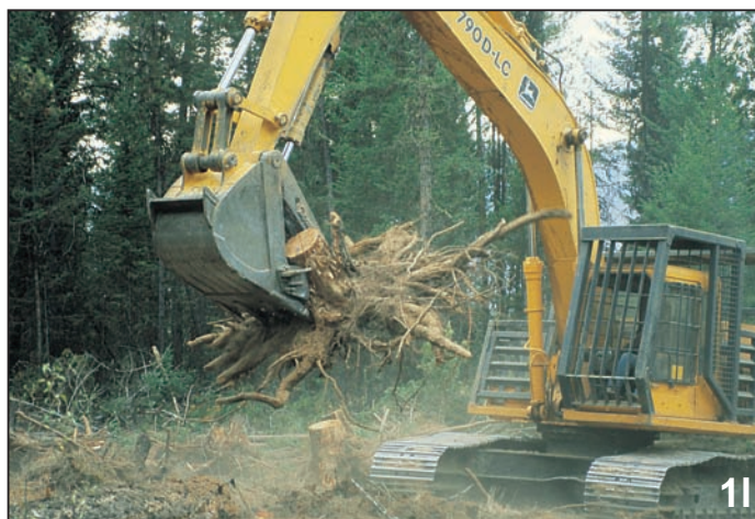
Figure 1j: Butt rot in Engelmann spruce. 1k: Transfer of A. ostoyae from a colonized stump to a living tree in a spaced stand. Figure 1l: Stump removal to reduce Armillaria inoculum.
