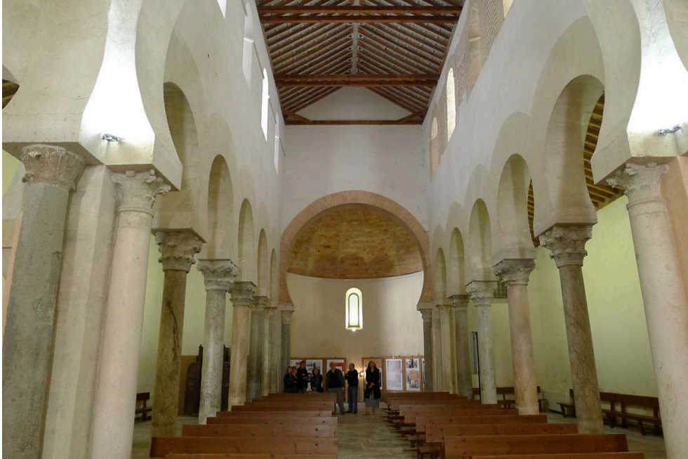
Fig. 4. San Cebrián de Mazote (Valladolid), regular keystones and reused and new elements of the internal arcades, looking westwards (cl. M. a Á. Utrero).
