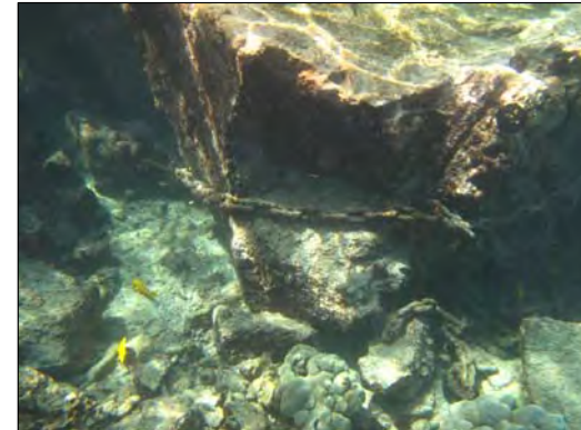
Figure 7. Old mooring chain around boulder.
