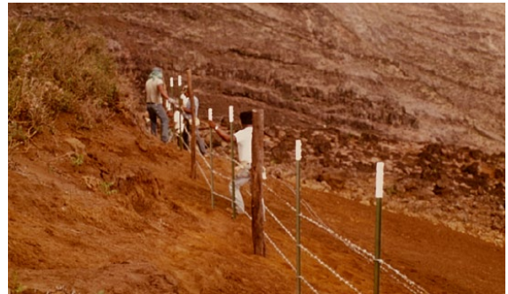
Figure 43. Fence construction in 1982
