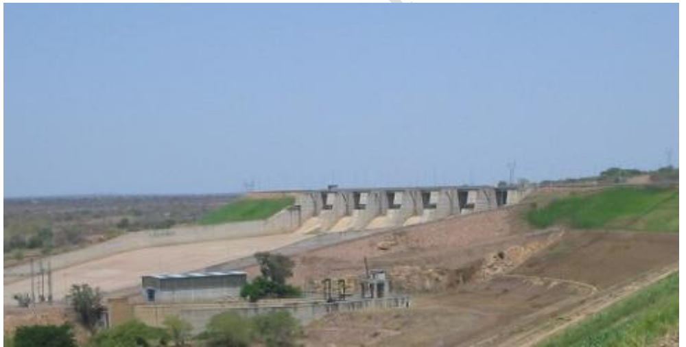
Figure 3-3 Corumana Dam. Dam piers on spillway crest and overhead concrete beam for installation of six radial gates were already constructed in 1983-89.
