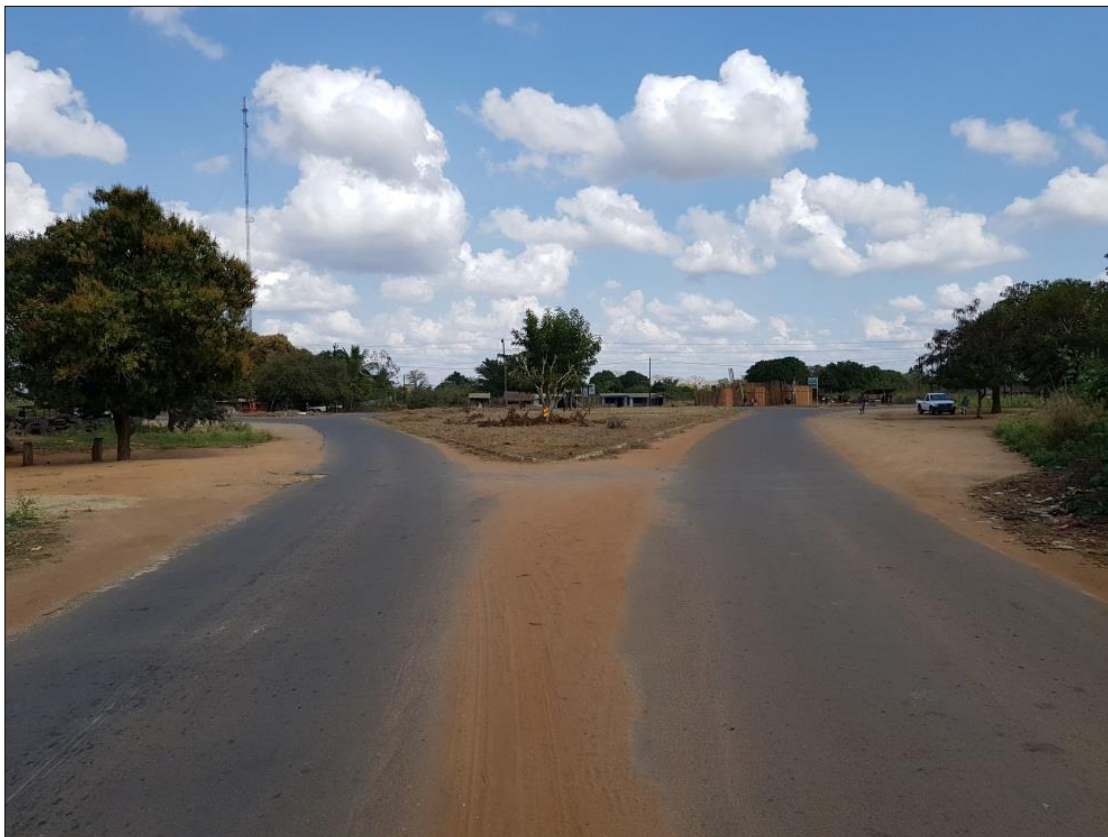
Figure 116: R241/EN1 Intersection: Eastern Approach
