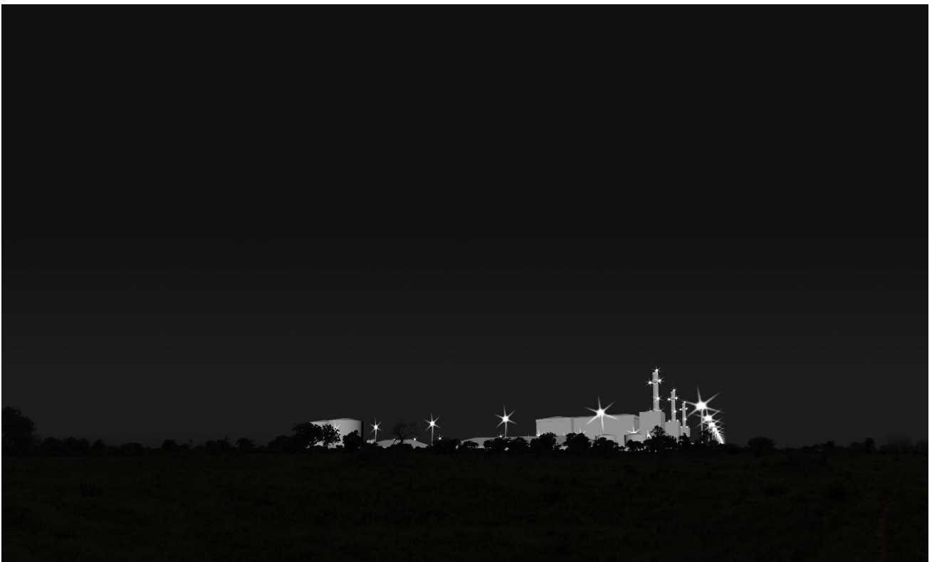
Figure 144: Light pollution at night from power plant (screened medium-range view)
