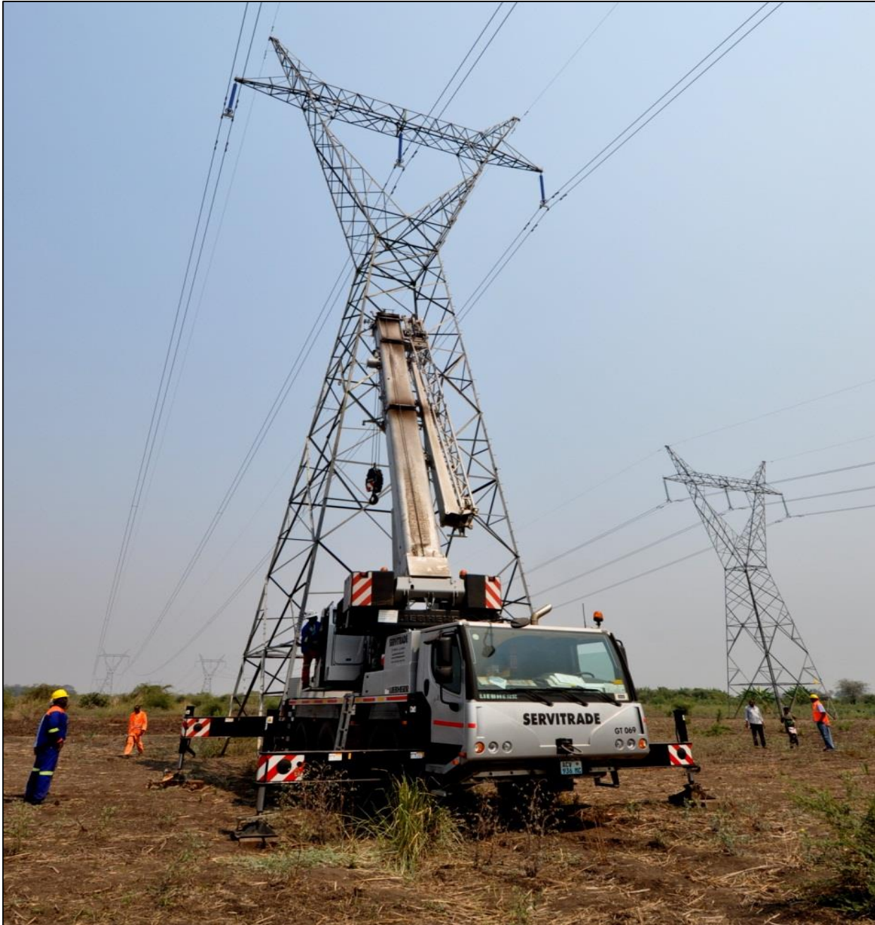
Figure 26: Example of Pylon construction (source: http://cscon.co.za/ and EDM)
