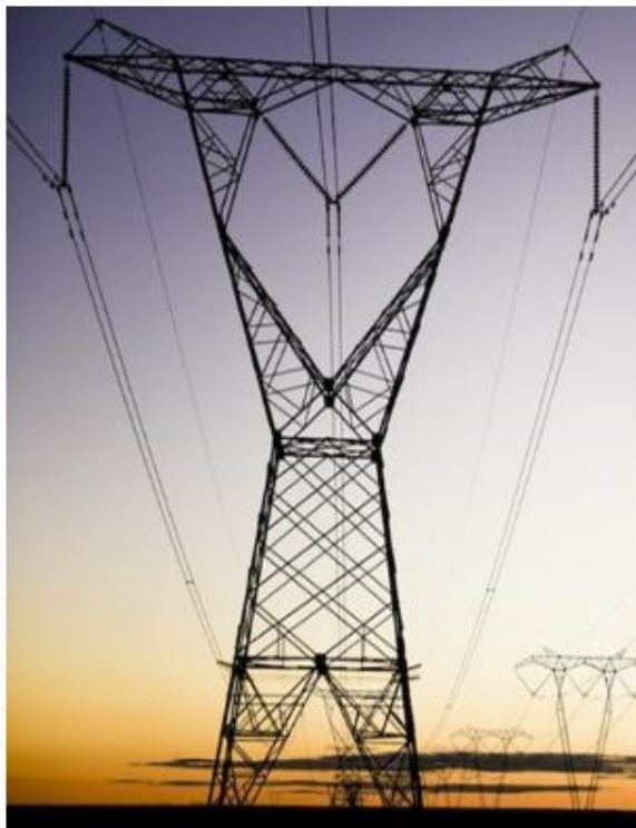
SUSPENSION TOWER - Y TOWER
