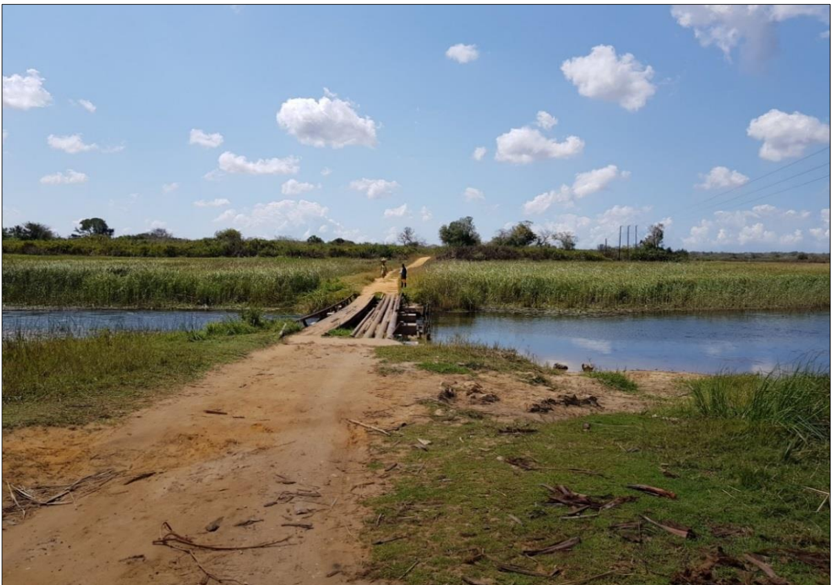
Figure 120: Shortcut road pipe bridge
