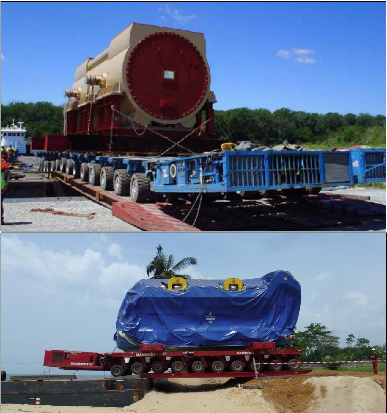
Figure 12: Example of large equipment being offloaded from a barge (Note the levels of the ramp, the barge and the jetty (source: SUBTECH))
