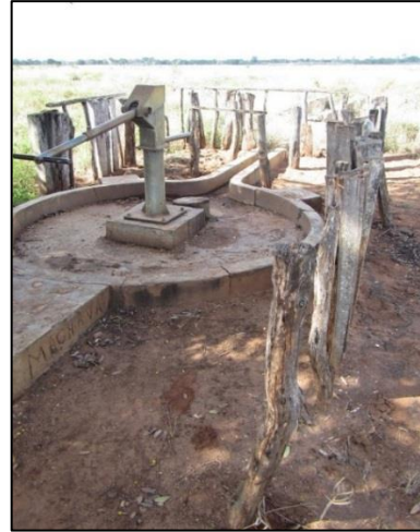
Figure 86: Hand pumps have been installed close to some villages to provide drinking water to local people
