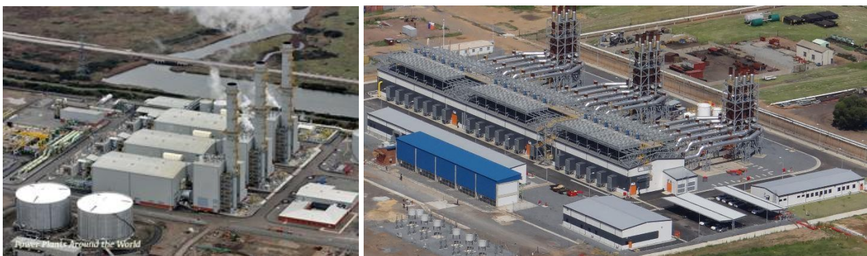
Figure 3: Examples of gas to power plant sites (source: www.industcards.com and www.wartsila.com )
