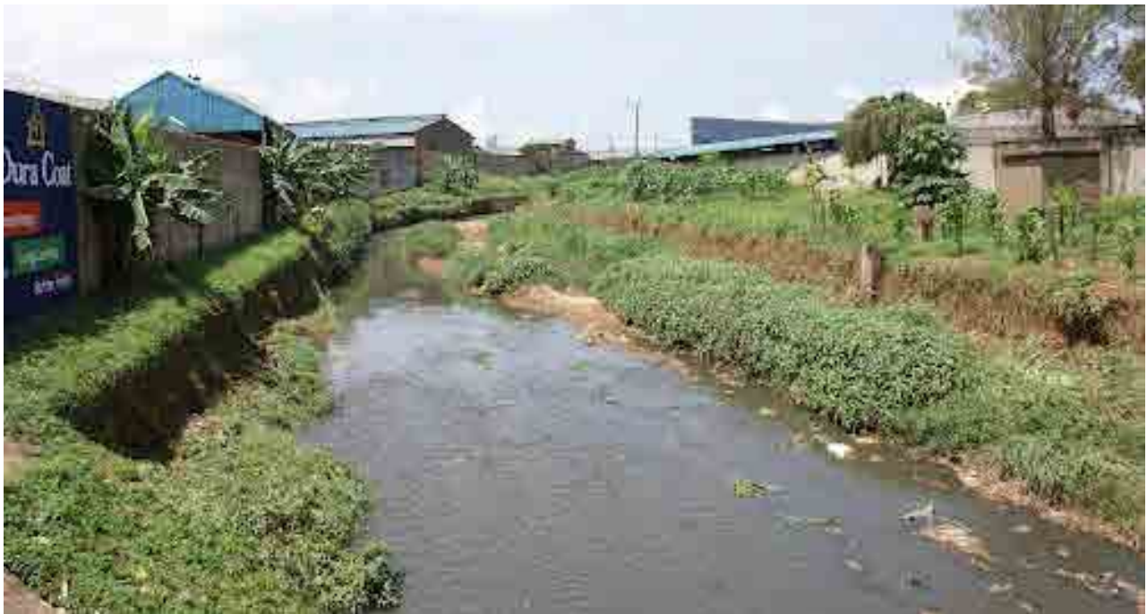
Figure A5.2 Nakivubo channel at 5 th Street Bridge
