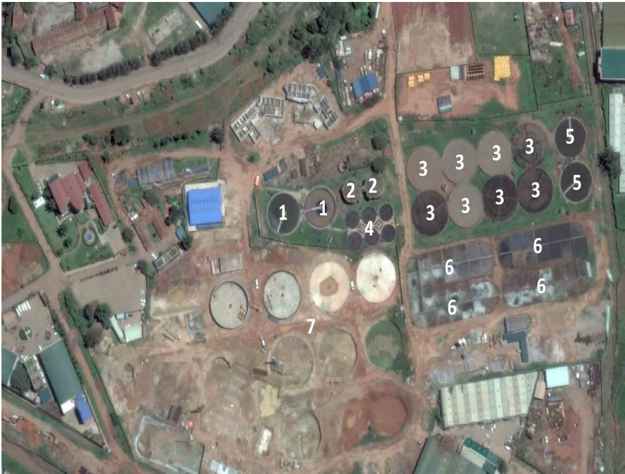
Figure A6.3 Bugolobi WWTW from Google Earth on 18 July 2015. The various unit processes indicated are as follows: (1) Primary Settling Tanks, (2) Digesters, (3) Large Trickling Filters, (4) Small Trickling Filters, (5) Secondary Settling Tanks, (6) Sludge Drying Beds, (7) Demolished structures, most probably old trickling filters.
